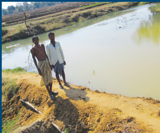
EARTHEN CHECK DAM
